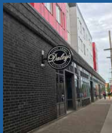
Daley's Restaurant, the oldest restaurant in Chicago, relocated across the street from its original site to a larger, more modern location. The restaurant is highly visible from busy Cottage Grove Avenue and 63 rd Street.
