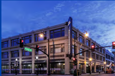
Award winner for Adaptive Use, the Aurora Arts Center contributes to downtown Aurora's revitalization while providing a space for artists to live and work.
