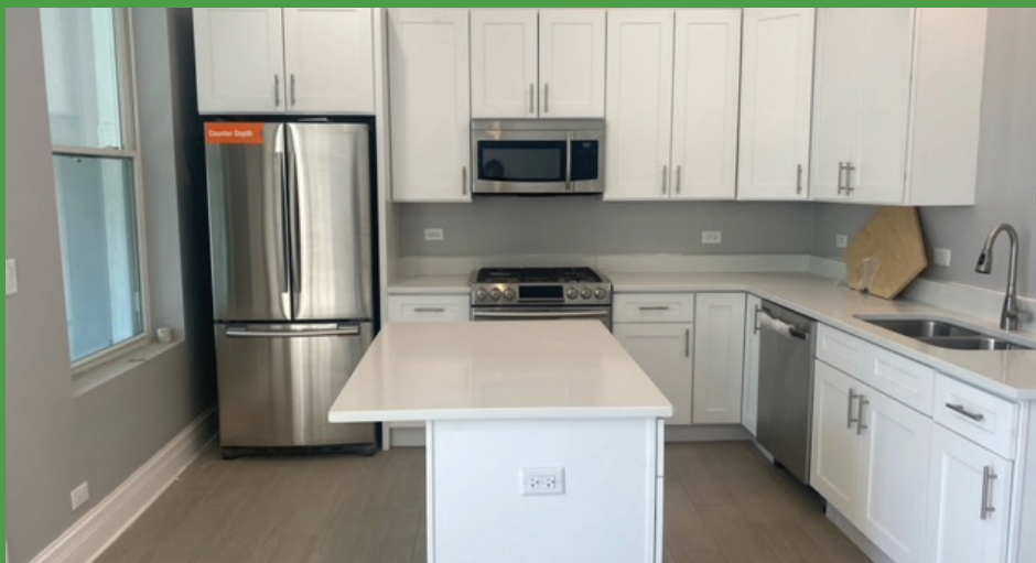
The West Garfield Park building on Gladys required extensive work. Washington installed new flooring, windows, and constructed a fully functional, modern kitchen.
