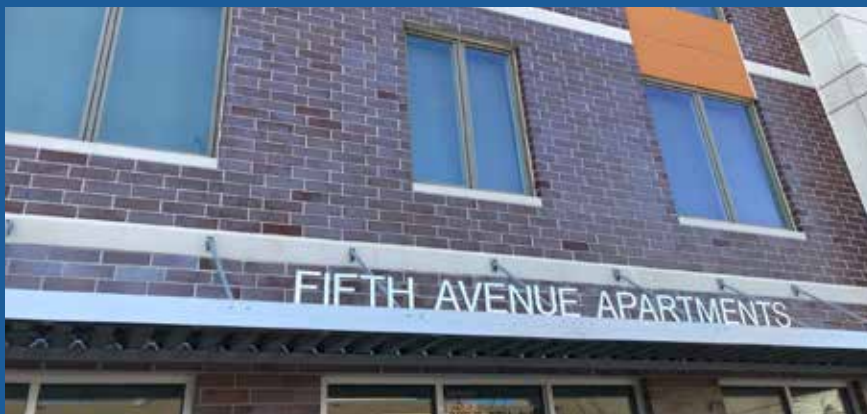
Common areas in Fifth Avenue Apartments are enhanced with expressive art statements and energy-efficient LED lighting.
