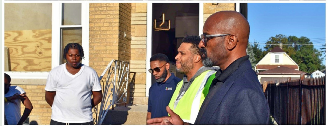
Top: Community developer, Levar Love; project crew, Telly Safford; Robert Raphael Moore; Tevin Merkson; Lordell Ratliff; Donnie Slaughter. Below: Donnie Slaughter, project crew; Sean Harden, CCLF consultant; Jason Martin, 1 City United; Will Edwards, Chicago Department of Housing.
